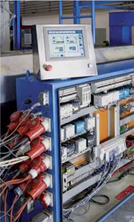
no kind of sequence mechanism or PLC logic function. The KS98-1 offers this functionality, but all within a DIN housing. And because it is still a DIN controller and not a PLC, the set-up of the process is more cost-effective. The customer's problem could have been solved with a PLC, but this would have also required the expensive services of a high-end PLC programmer with a lot of knowledge.
